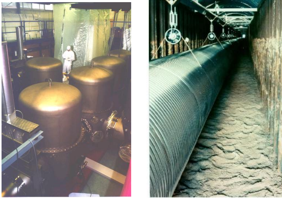
Figure 1. The buildings of GEO 600 are split into three regions with different cleanroom classes: The so-called gallery where people can work with normal clothes, the inner section which has a cleanroom class of 1000 and a movable cleanroom tent installed over open tanks with a class 100 cleanroom. The convolute beam tube has a diameter of 60 cm and a wall thickness of 0.8 mm. The tanks are 2 m tall and accommodate the triple-pendulum suspensions of the interferometer mirrors.
