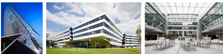
Figure 2.3: Examples for the application of intumescent coatings. Left: Post Tower Bonn (built in 2003, photo: Claus Boeckh), middle: Adidas Laces Herzogenaurach (built in 2011, photo: kadawittfeldarchitektur) and right: The Squaire Frankfurt (built in 2011, photo: fylo)
