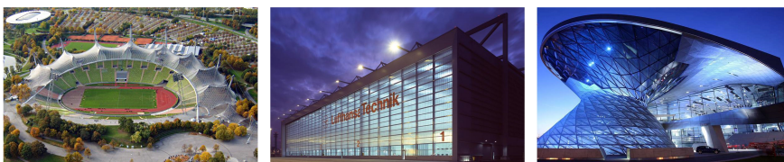
Figure 2.2: Examples for the application of intumescent coatings. Left: Olympia Stadium Munich (built in 1971, photo: Olympiapark München GmbH), middle: Maintenance Hangar Lufthansa Frankfurt (built in 2007, photo: gmp Architekten) and right: BMW World Munich (built in 2010, photo: Getty Images)
