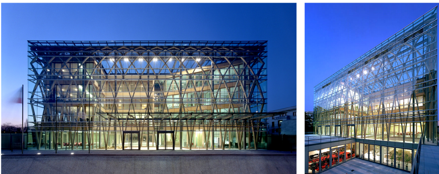
Figure 1.1: Government building of North Rhine-Westphalia with a glass facade and a steel structure with an intumescent coating that ensures a fire resistance rating of 30 minutes (built in 2002, photo: pinkarchitektur)
