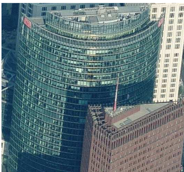
Figure 8. Oblique view aerial image of the DB-Tower
