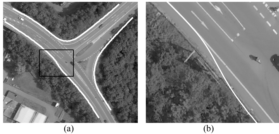
Figure 4-19: Incorrectly extracted road border. Marked box in (a) shows the area where inconsistency occurs. This area is displayed in detail in (b).
