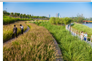
A1.4: Submersible vegetation A2.1: Reshaping the floodplain with more gently sloping banks A3.1: Terraced bank
