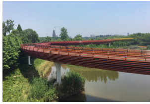
A4.3: Bridge over the water
