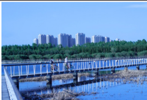
A4.5: Raised boardwalks and platforms
