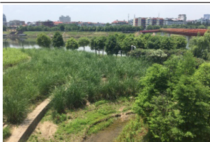
A1.4: Submersible vegetation A2.1: Reshaping the floodplain with more gently sloping banks A3.1: Terraced bank
