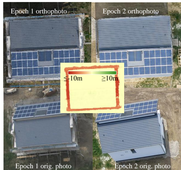
Figure 4: Dismantled scaffolding around a building
