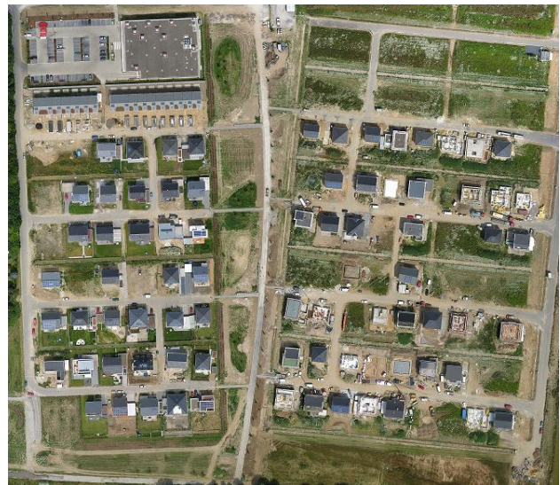
Figure 1: Orthophoto of the zero:e-park acquired in the monitoring campaign (processed by PhotoScan)
