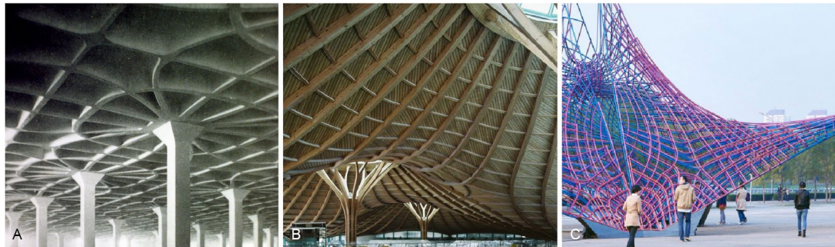
Figure 1: Architectural designs using the Principal Stress Directions.
