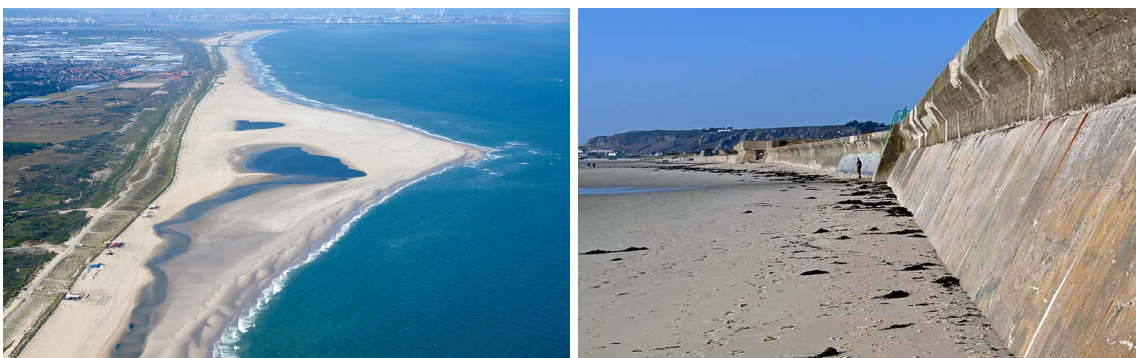
Figure 1.1: Shoreline protection against erosion. Left: Mega beach nourishment (sand motor), the Delfland Coast, the Netherlands ( https://dezandmotor.nl/fotos-en-videos/ ). Right: Seawall at La Crabriere, St. Ouen's bay, Jersey, Photo: Oliver Dixon.
