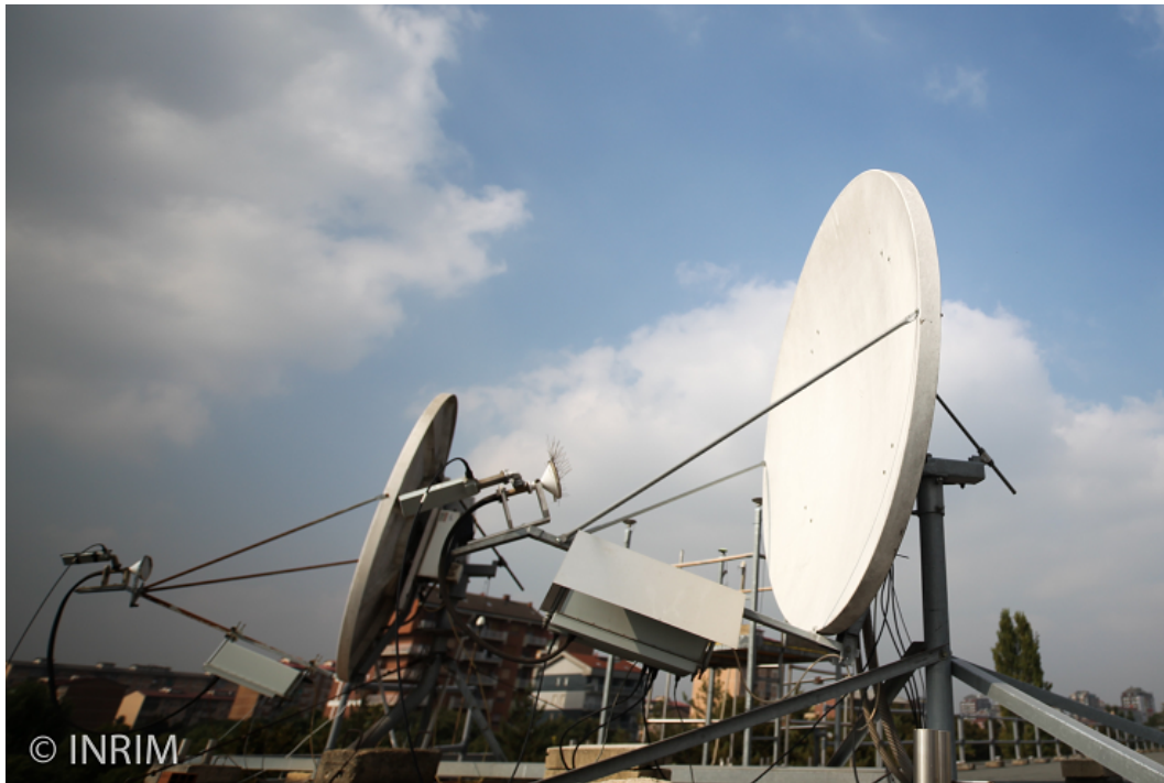
FIGURE 2.7: The roof station at INRIM (Istituto Nazionale di Ricerca Metrologica, Torino, Italy), with a transceiver attached to the antenna which comprises an amplifier for the outgoing signal and up- and downconverter. By courtesy of INRIM.
