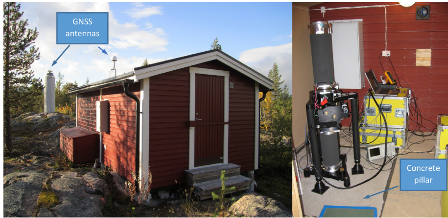
Figure 2. Example of a typical AG station: Arjeplog, Sweden (ARJE).
