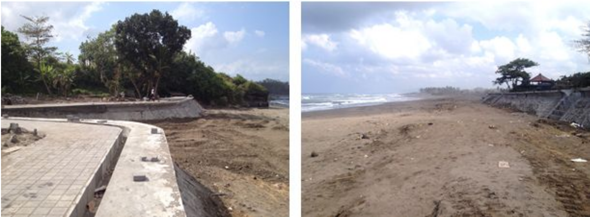
Fig. 6 Hard-structure seawall in Tabanan, Bali © David,2014
